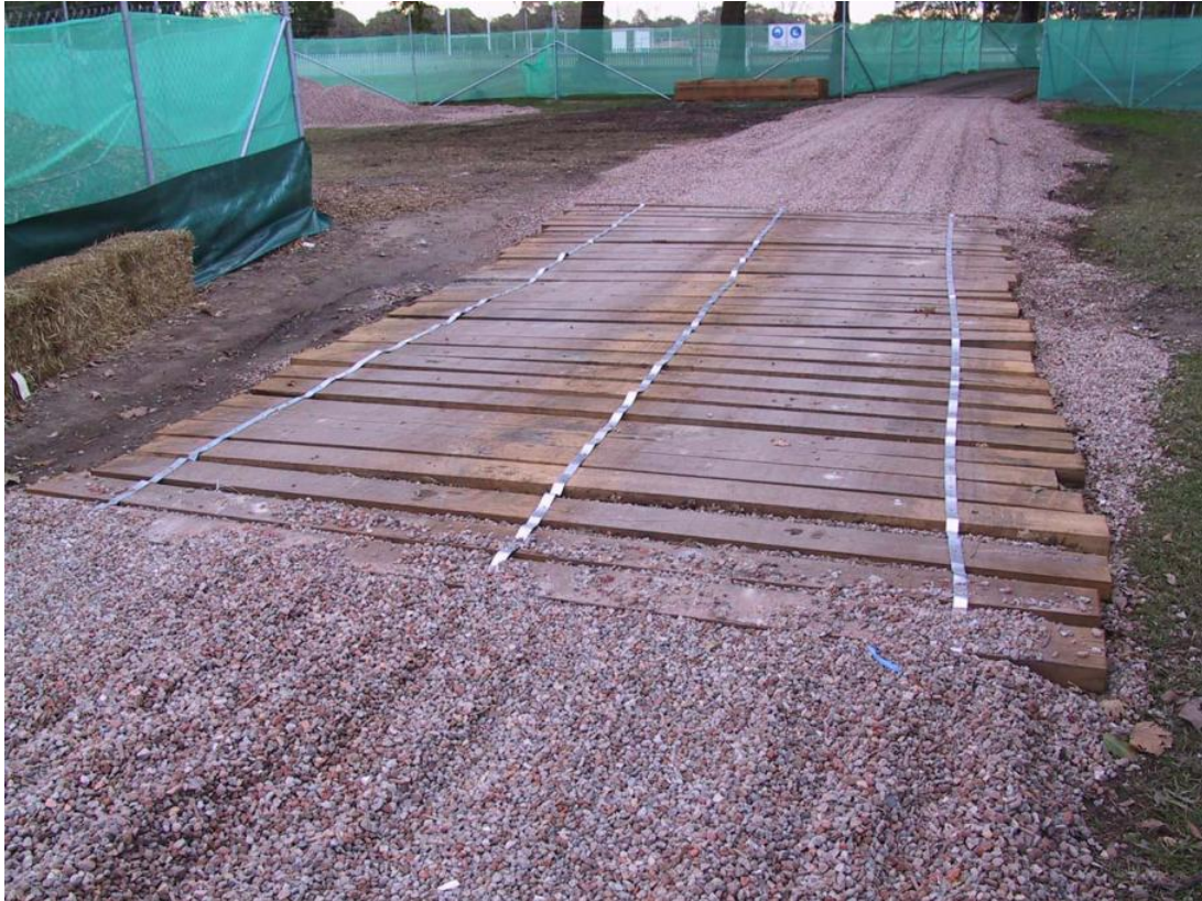
Figure 11 – Example of acceptable Tree Protection Area ground protection
