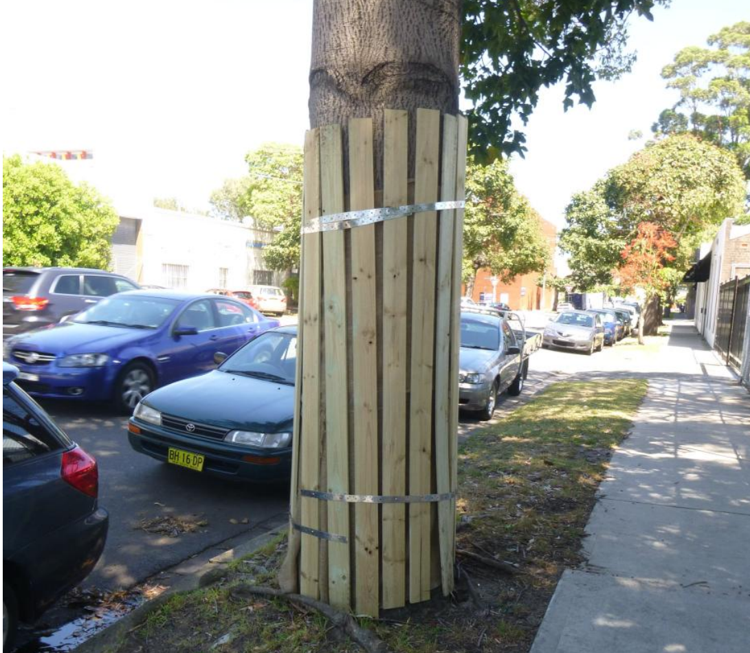
Figure 12 – Example of acceptable Trunk Protection batten installation
